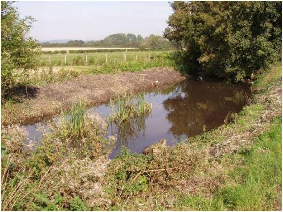
Ratham Lane section cleared
