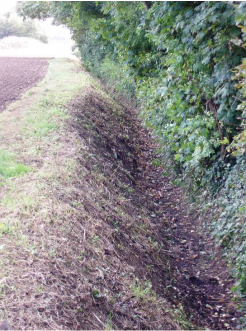
East Ditch cleared
