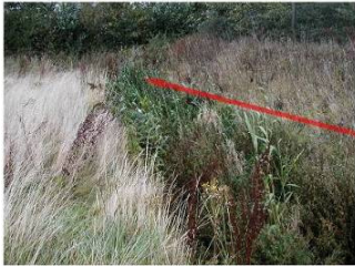
Exit ditch from Brinkmans Blocked
