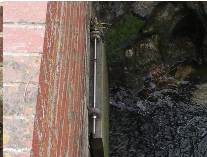
Afterwards with SS rod and locknuts
