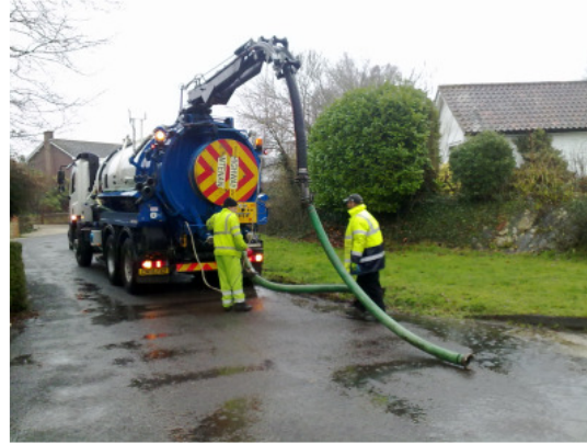
WSCC Jetter in Crede Lane
